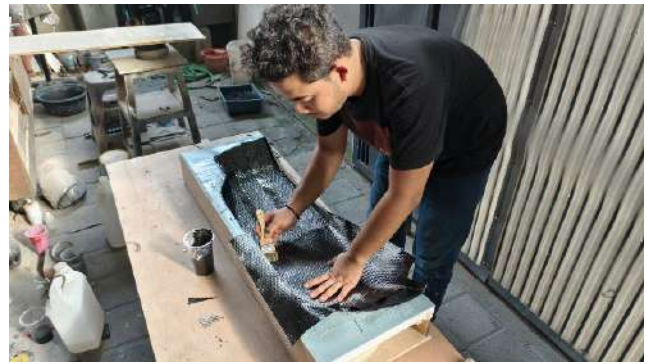
Fig. 12. Hull production process
