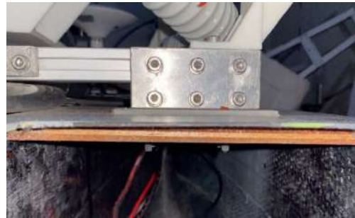
Fig. 17. Main deck base installation
